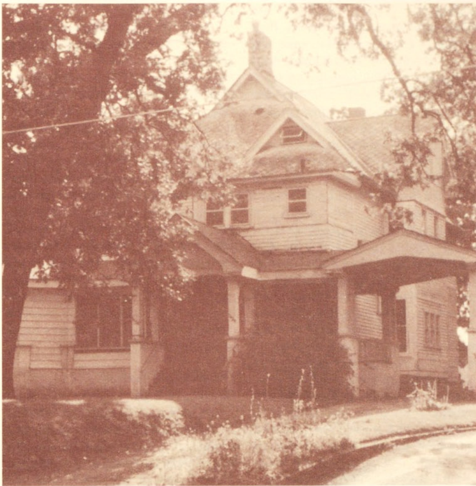
Still standing but not in the best of condition is the Ladd family home on the near north side of Des Moines.
