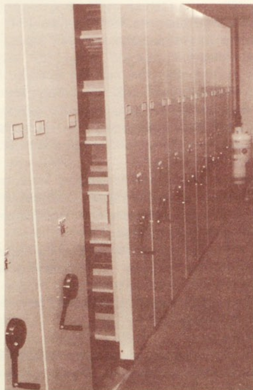
Inside the new climate-controlled vault with its compact storage units. A walk-in cooler in the rear keeps video and audio tapes at low temperature and humidity.
