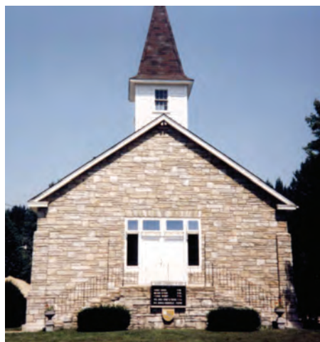
The front of Keene Assembly of God, during renovations, 1987.
