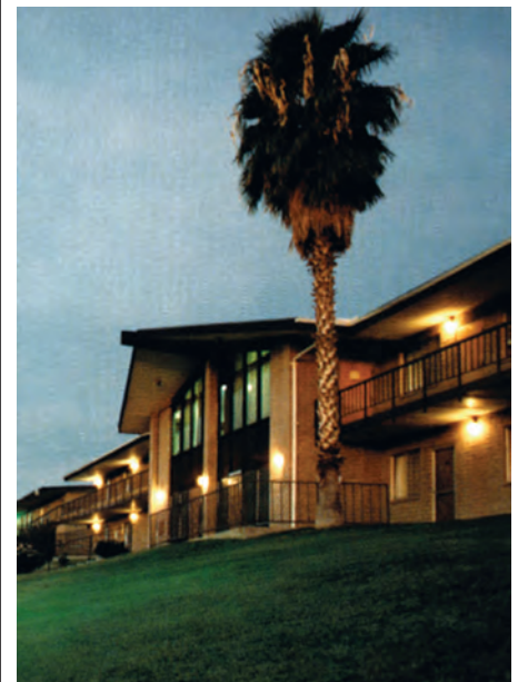
The Alta Washburn multi-purpose building at American Indian College, Phoenix, Arizona.
