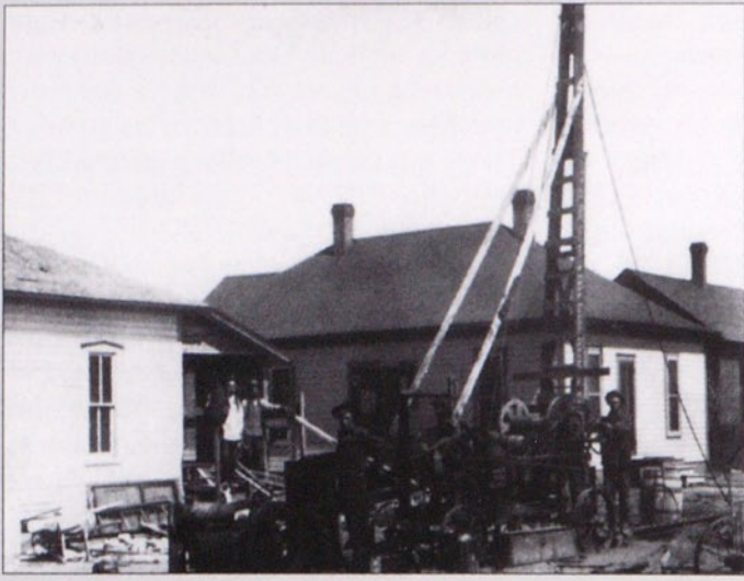
Henry Krause, the future plow manufacturer, using a well-drilling rig about 1907. He is standing in the center.
